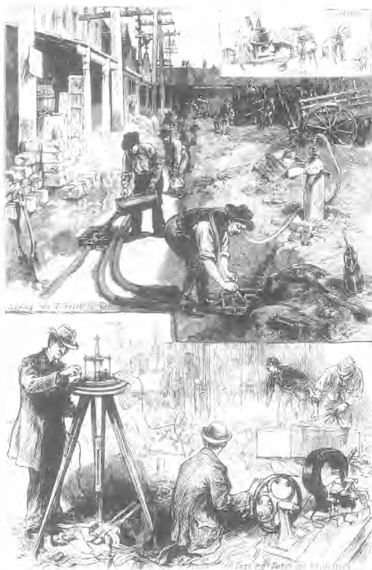
FIG. 10. A "Harper's Weekly" illustration of the laying of the original Edison underground mains in New York, U.S.A. These supplied electricity over a square mile of Manhattan from the Pearl Street generating station in 1882.
